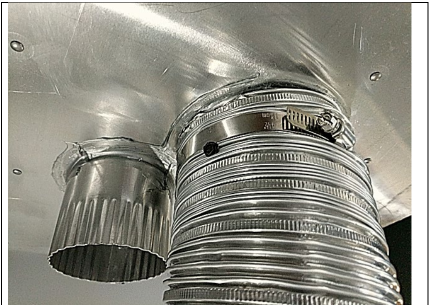
Vent Cap Flex Connection Hose Clamp first. Secure w/ Screw below Hose Clamp
