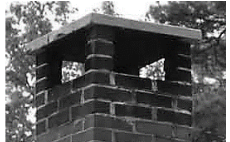
Concrete Cap Chimney Top
